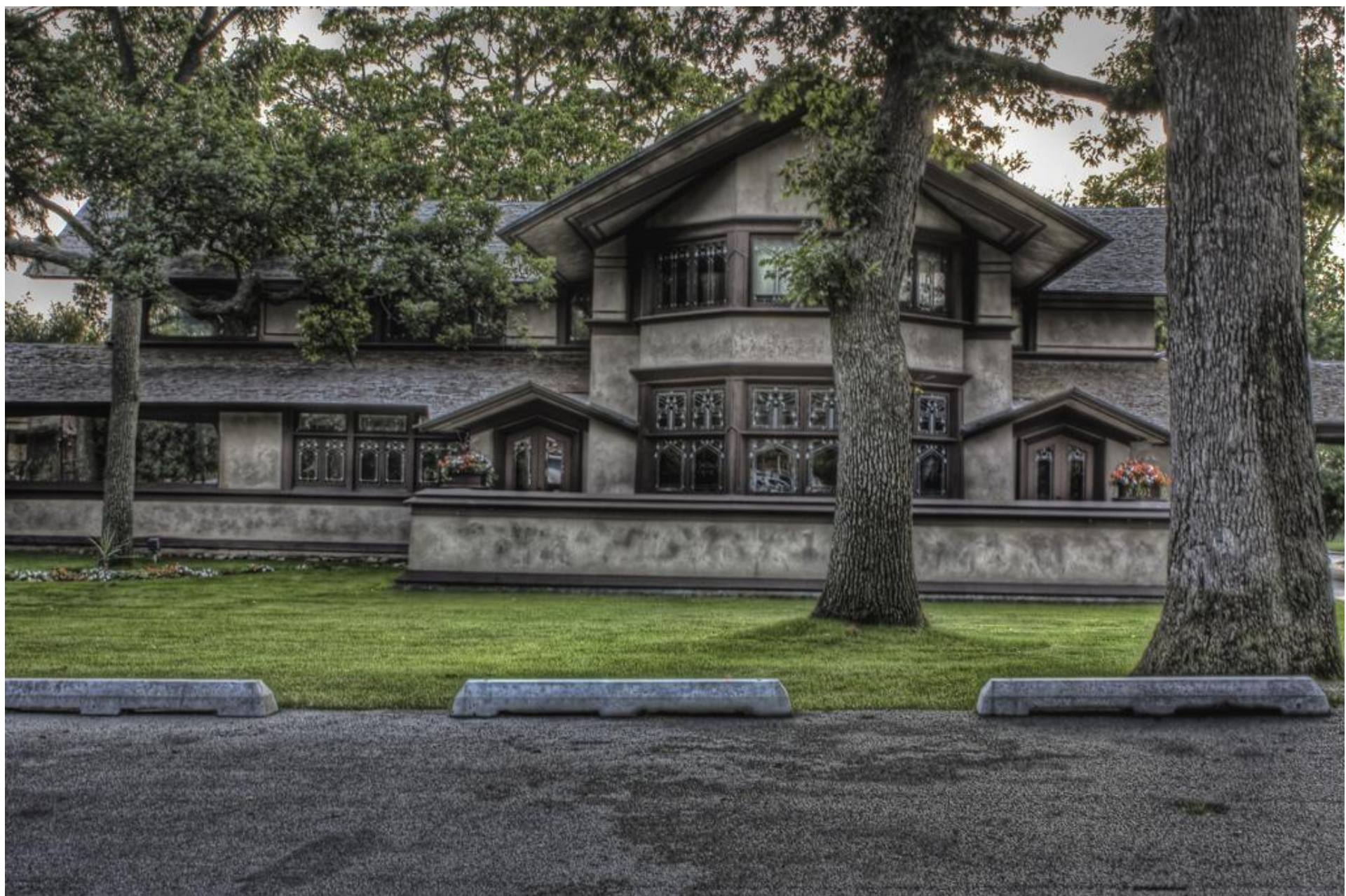
Harley Bradley House
