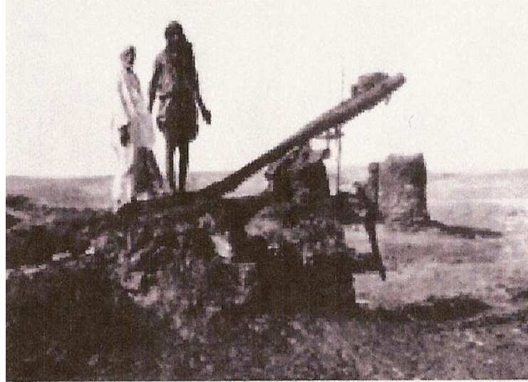
A primitive well baling device for raising oil from seeps. Once raised the oil was run into a small settling tank (dark oblong, right foreground)
