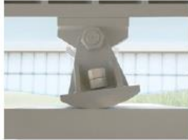
The rocker support for this bridge girder allows horizontal movement so the bridge is free to expand and contract due to a change in temperature. (4)
