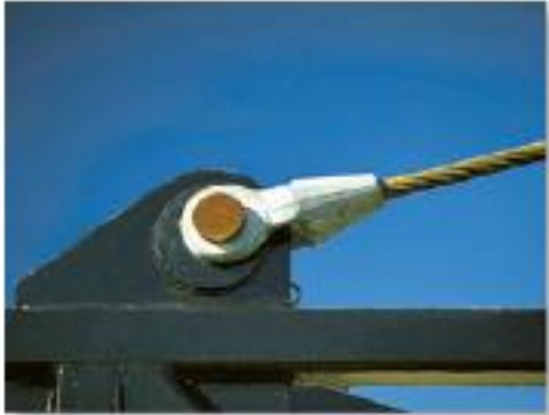
The cable exerts a force on the bracket in the direction of the cable. (1)
