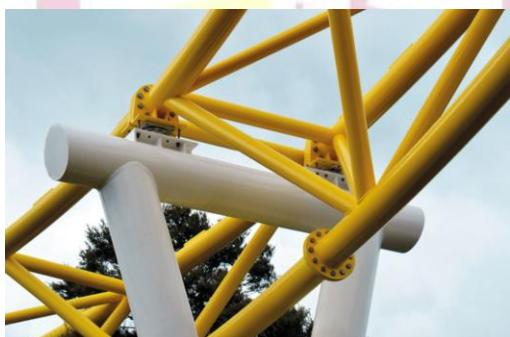
End plate connectors have been used to attach the long triangular truss sections of this pedestrian bridge in Auckland, New Zealand.
