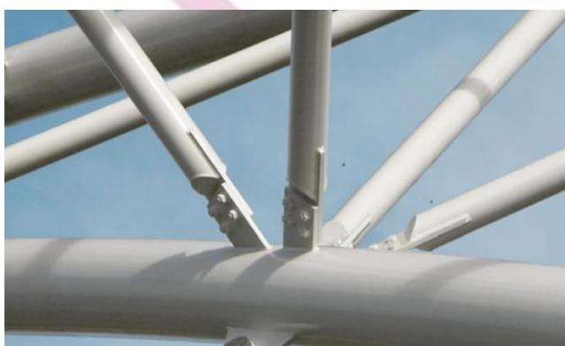
Bolted connections with simple lap joints constitute the internal connections in this pedestrian bridge truss.
