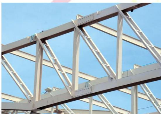
This 76m/250ft-long truss uses **bolted splice plates** in the top and bottom. The diagonal ladder-like web member was bolted into place at the time of splicing.
