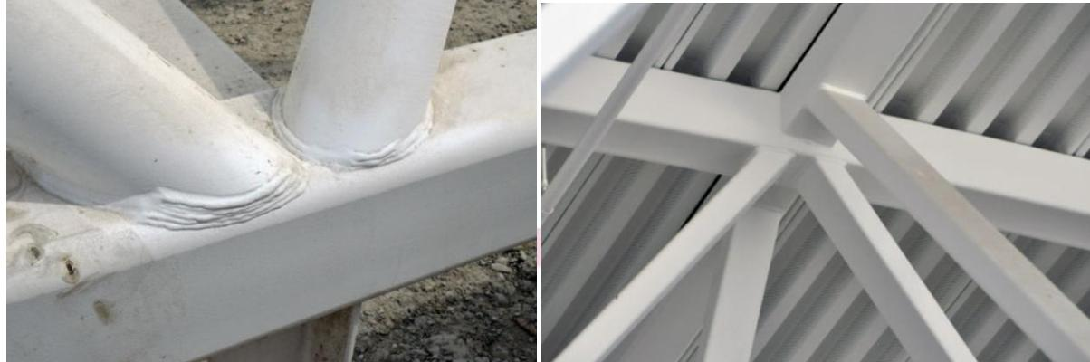
Tube-to-tube connections become more complicated when it is not possible to use a straight-angled cut to create the joint.
