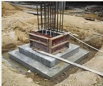
Isolated Footing (Single Footing)
