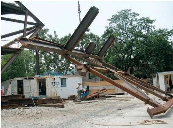
Left: The crane attachment for a truss element
