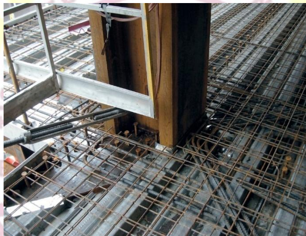
Prior to pouring the concrete floor slab.
