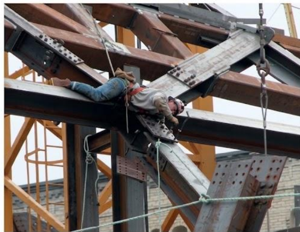
Right: The lead ironworkers resolving a steel connection issue
