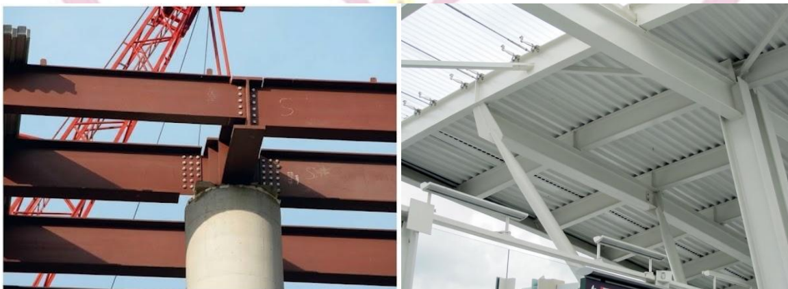
Beam -to-Girder Connections
