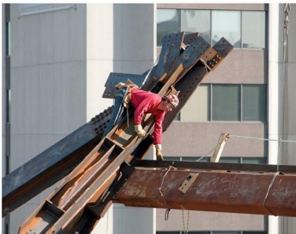
Left: Ironworkers guide a large steel beam into position.
