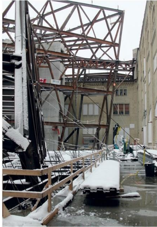
Work proceeds on the ROM during the winter months
