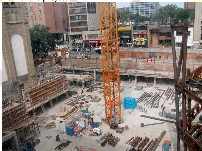
The location of the single-tower crane
