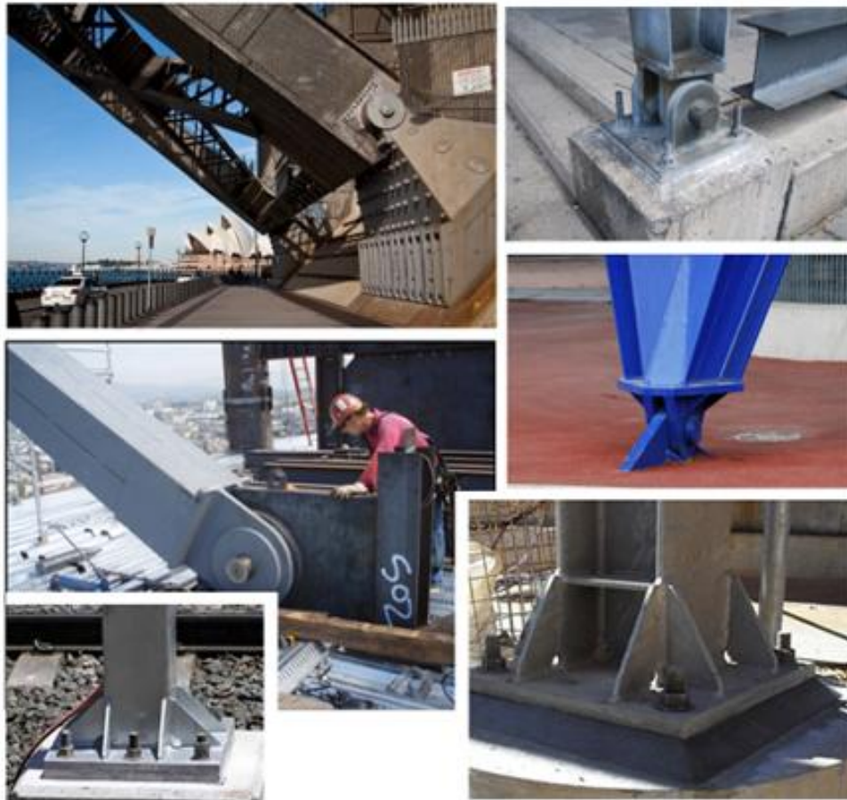
Columns End restraint
